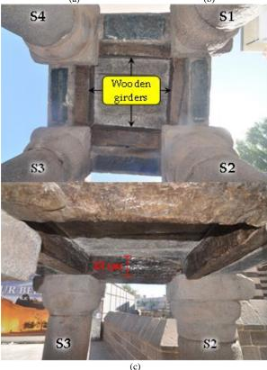
**Figure 3.** Photographic view of: (a) four cylindrical columns (west view), (b) brick girders (west and north views), and (c) wooden girders (bottom view)
