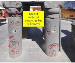
**Figure 10.** Photographic views of damages caused by firearms on: (a) the body and (b) columns of the Four-Legged Minaret (taken in 2021)
