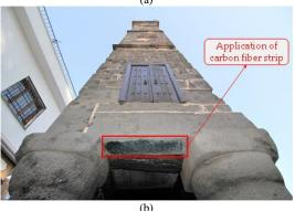
**Figure 5.** Photographic view of strengthening work on the Four-Legged Minaret: (a) application of steel clamps (taken in 2015) and (b) application of carbon fiber strip (taken in 2021)
