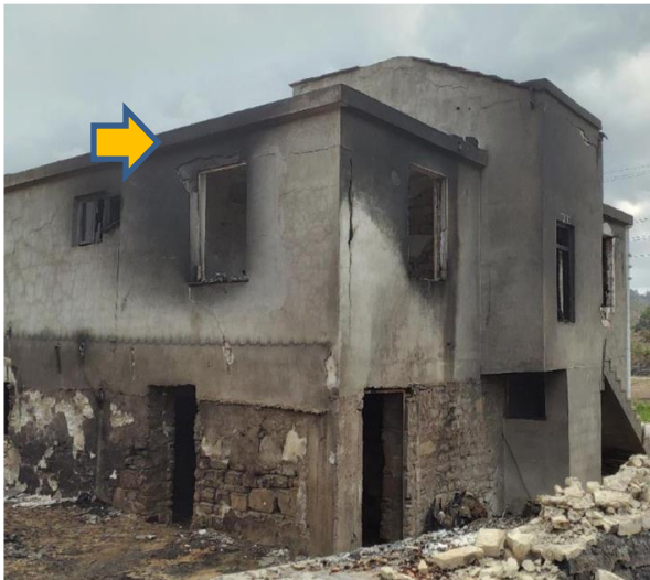
Figure 13: Reinforced concrete slab roofs (a and b)
