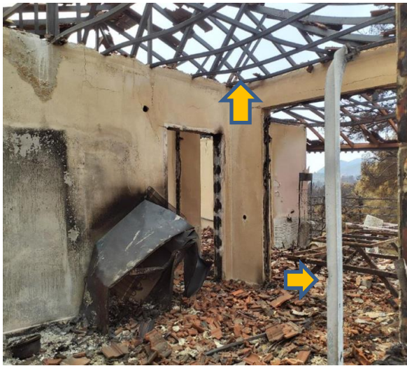
Figure 15: Light steel roofs-totally destroyed ( a and b)
