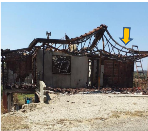
Figure 14: The timber on steel roofs- totally destroyed (a and b)
